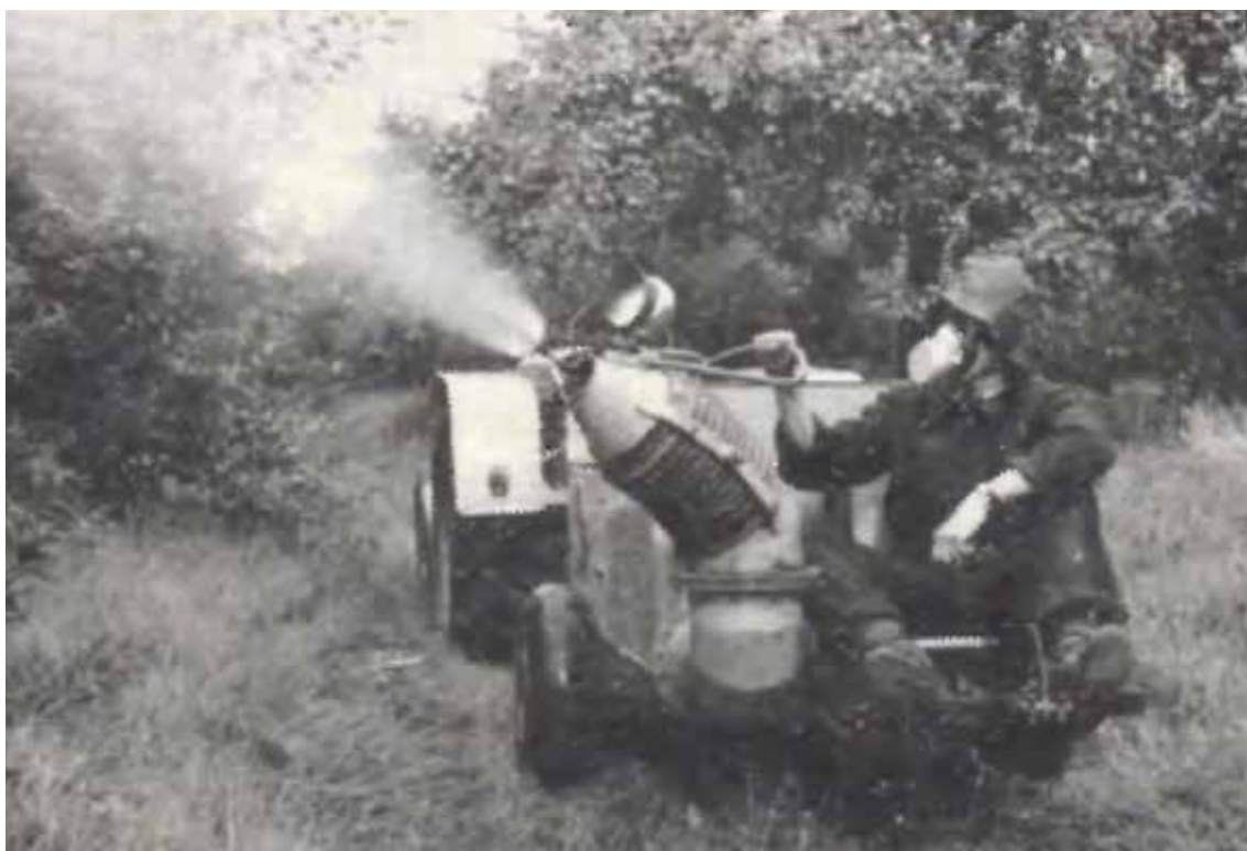
Afb 32: Motornevelspuit, 1954 (Lit. 31, p127)
